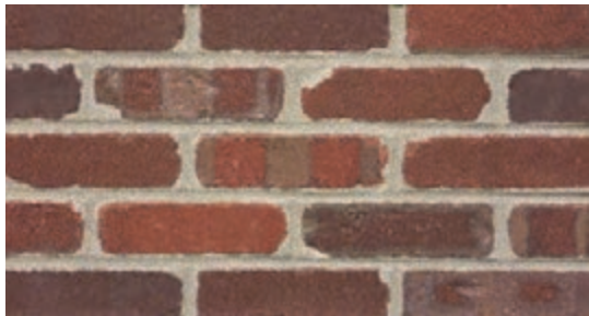
Standard 3/8" Mortar Joint
